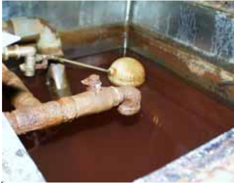
before installing Ion Water
